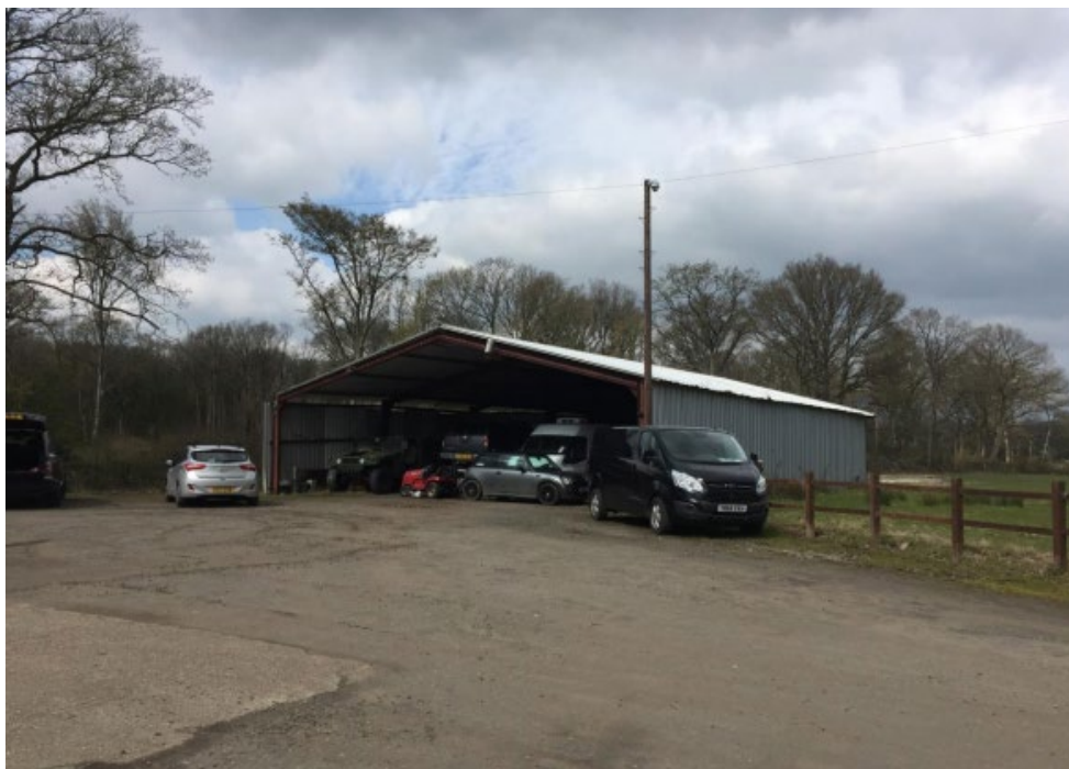
Figure 7: Existing Building (Open Fronted Barn C)
