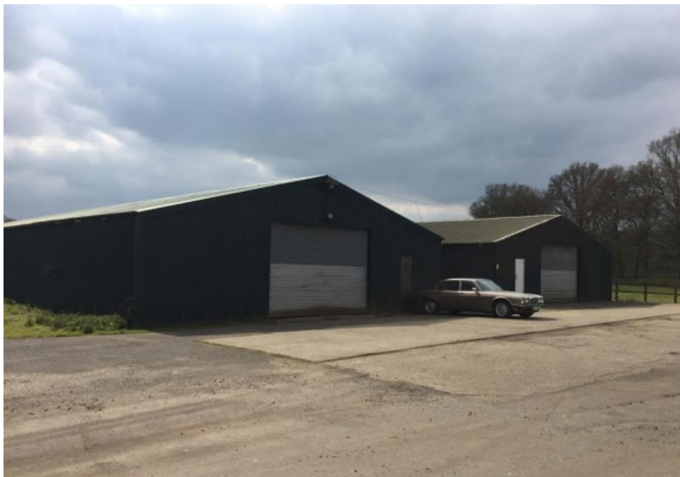
Figure 6: Existing Buildings (Enclosed Barns A and B)
