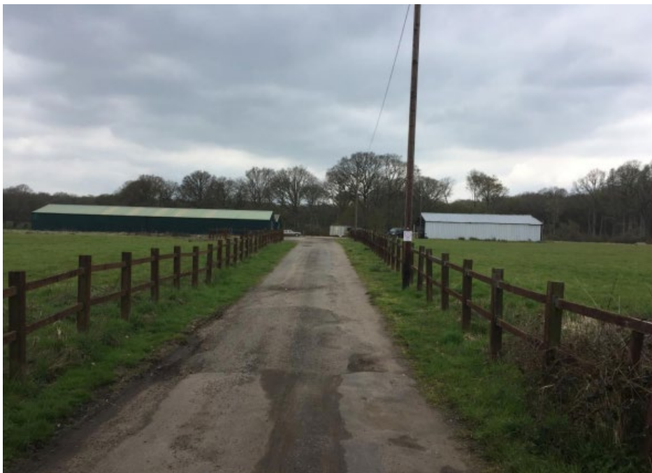
Figure 5: Existing Buildings from Entrance (Barns A and B on Left and Barn C on Right)
